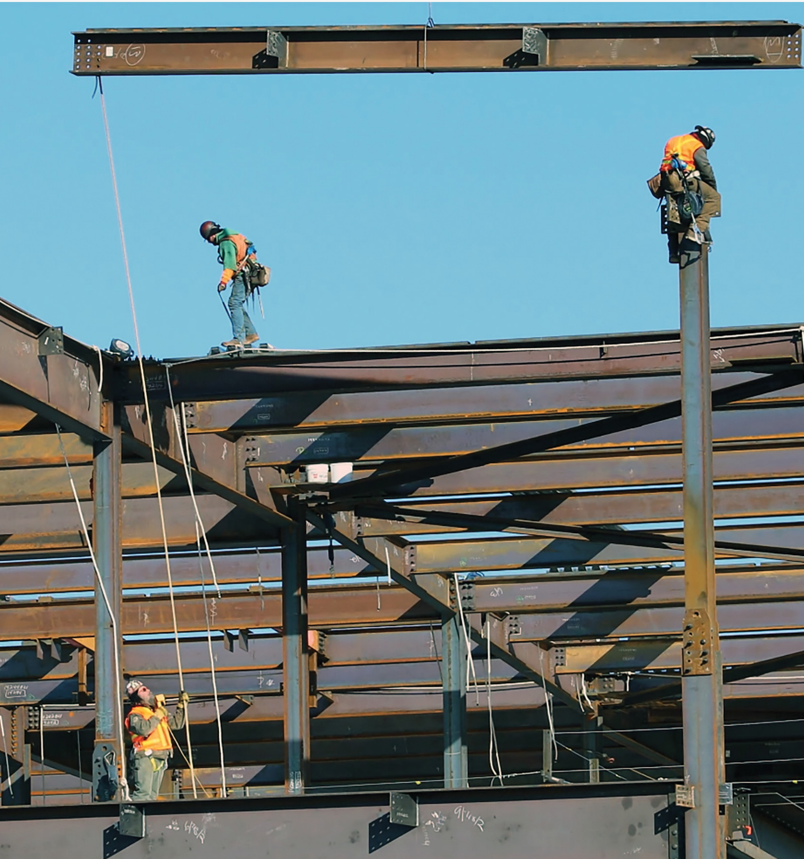
Construction workers at John F. Kennedy International Airport guide a steel beam into place.
