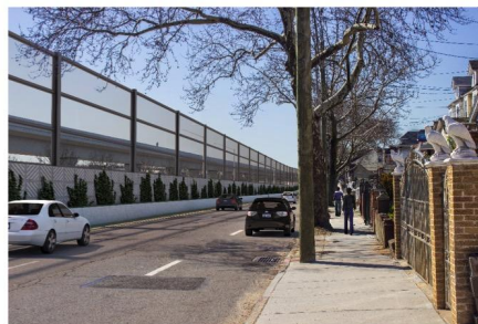
Proposed view of southbound service road between 105 th Avenue and 107 th Avenue
