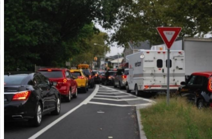
Existing view of northbound exit ramp to Linden Boulevard
