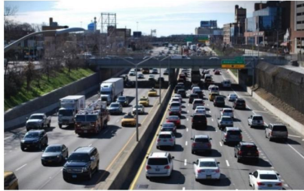
Existing view of VWE looking south from Hillside Avenue
