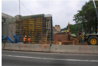
Construction of new retaining wall
