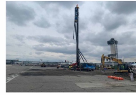
Pile Driving at Concourse A Site
