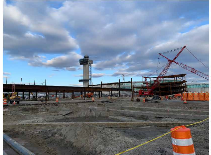
Concourse A Steel Erection
