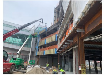
Concourse A Slab on Building Enclosure
