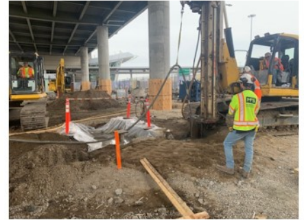
Headhouse Pile Driving
